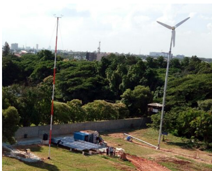
Fig.15 10 kW WiSH system at Renewable Energy Farm, Kodihalli Campus.
