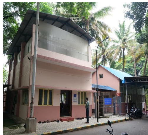
Sumukha Hall ( adjoining Ganesh Temple)
