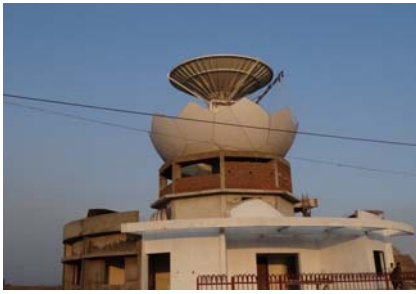
Fig. 19 The radome panel assembly in progress at Cherrapunji.
