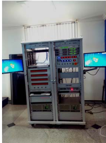
Fig. 20 IGAPS integrated with the automated test station.
