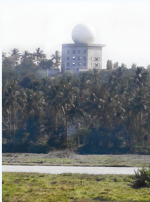
DWR Radome at Gopalpur, Odisha.
