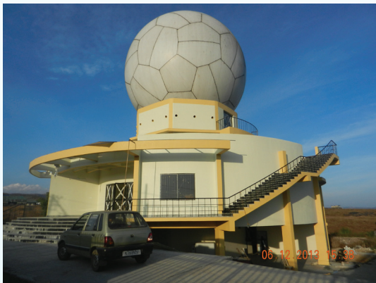
The 12.88m dia. DWR Radome installed at Cherrapunji, Meghalaya.
